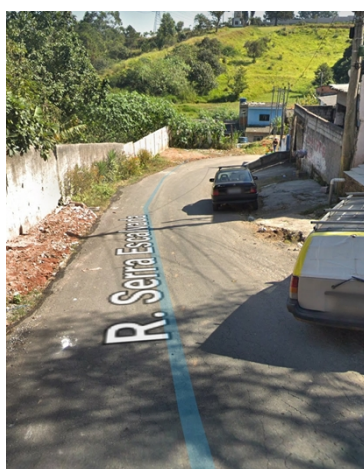
Rua Serra Escalvada
